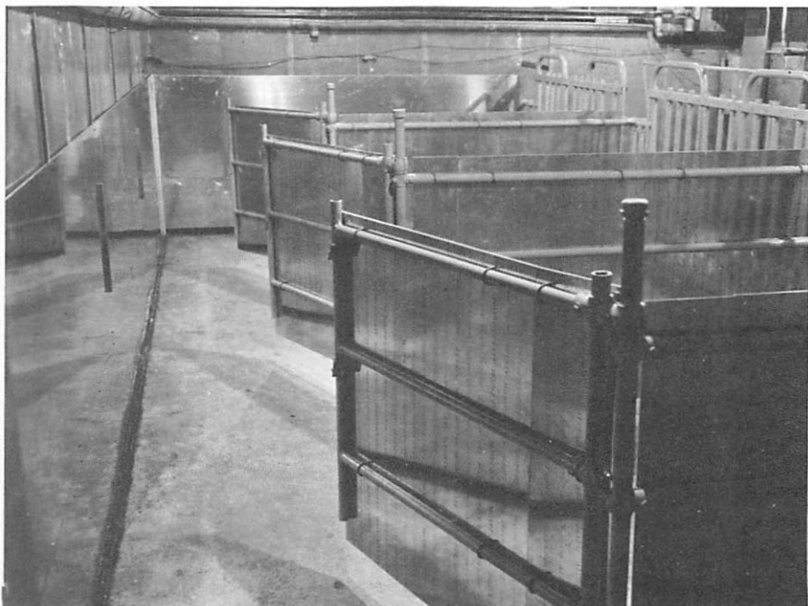
Fig. 2—Photograph of the calf pens within Test Room II. Aluminum, 3/16 inches thick, was placed along the three sides of the pens primarily for the protection of the walls and to isolate one pen from the other more completely. Ventilation air was discharged, horizontally, at near ceiling height from above the feed alley toward the rear wall (from right to left on the picture).
